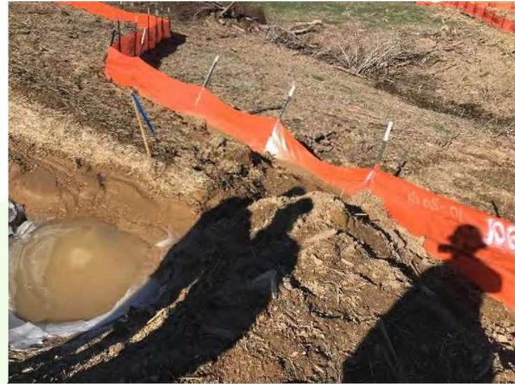
Accumulation of water overtopped ditch, eroded embankment, and damaged silt fence. Ditch and pipe not installed or maintained to ensure positive drainage to Basin 5-3.
