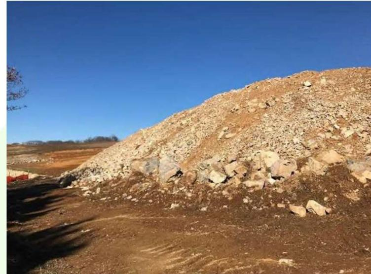
No stabilization measures applied to stockpile. No temporary silt fence.
