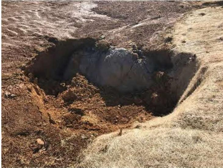
Sinkhole in Basin 3-3. Basin not maintained to hold the required wet volume per the Erosion and Sediment Control Regulations and the approved plan.
