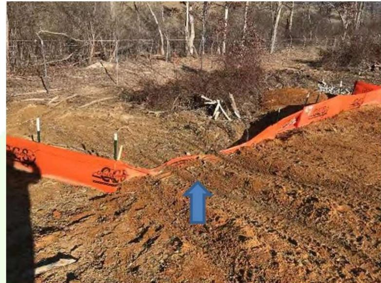
Silt fence behind Basin 3-3 not maintained in an effective operating condition.
