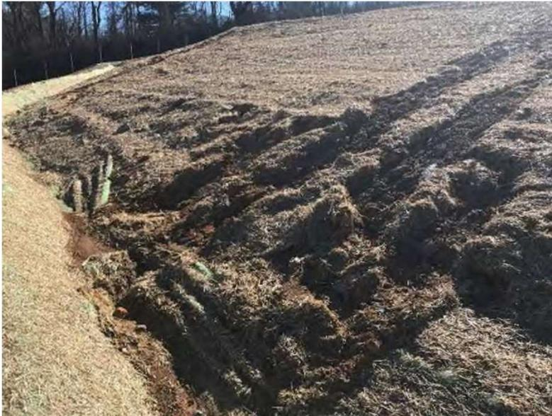
Erosion on slope above Ditch 5-3 East resulted in accumulation of sediment, decreasing capacity of ditch. Ditch not cleaned out.
