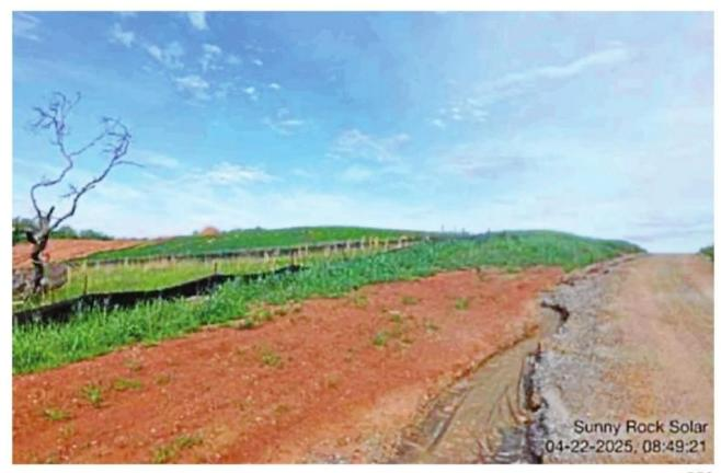
The DEQ reported concentrated runoff has resulted in channel erosion adjacent to the access road located across from Memory Lane in a report of Sunny Rock Solar LLC.
