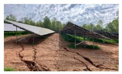
This photo from a Virginia Department of Environmental Quality inspection report from April shows what the DEQ said is erosion under solar panels at Sunny Rock Solar in Henry County. The erosion contributed to sediment being washed into nearby streams and wetlands, according to the DEQ.
