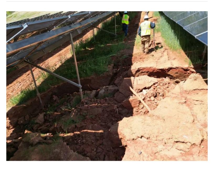
This photo from a Virginia Department of Environmental Quality inspection report from April shows what the DEQ said is erosion under solar panels at Sunny Rock Solar in Henry County. The erosion contributed to sediment being washed into nearby streams and wetlands, according to the DEQ.
